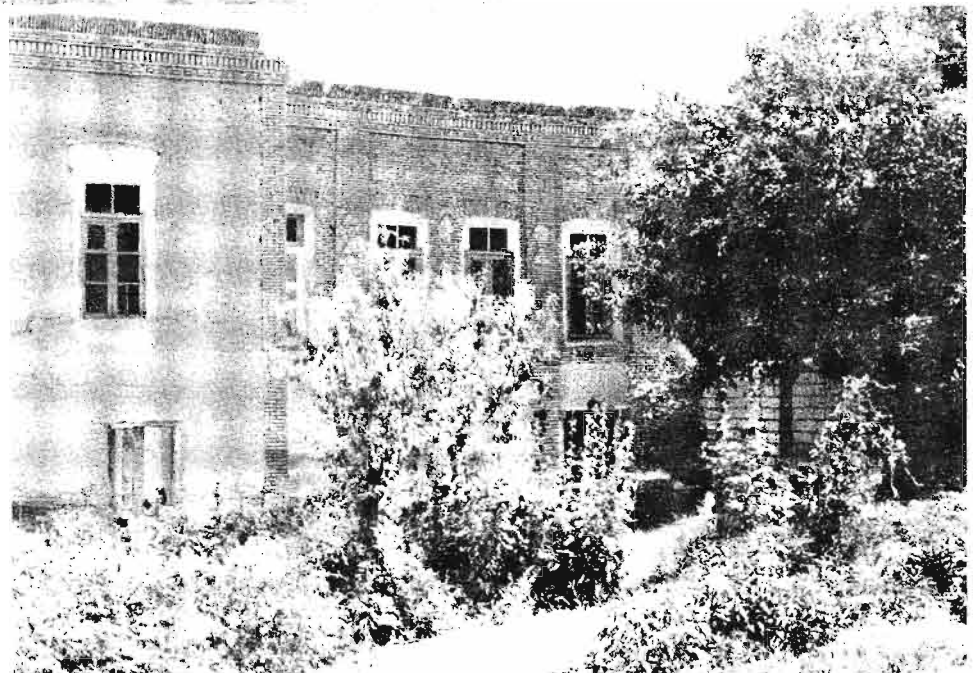
View from back showing courtyard
